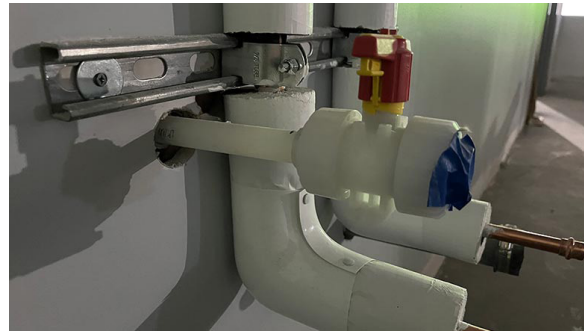
Food and research laboratory installation using PVDF pipe. Photo courtesy of Mtech Mechanical
